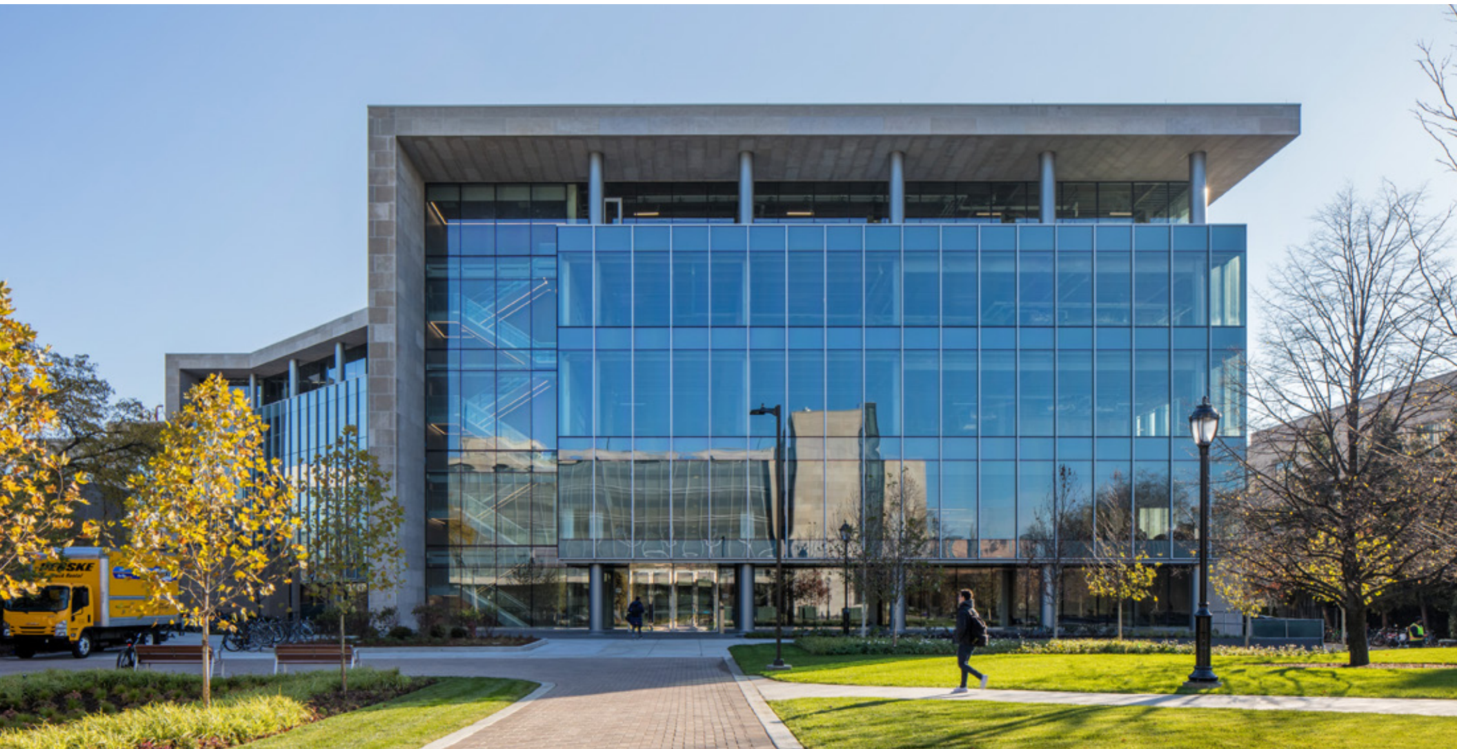
SCIENCE AND ENGINEERING LIBRARY AND LABORATORIES
