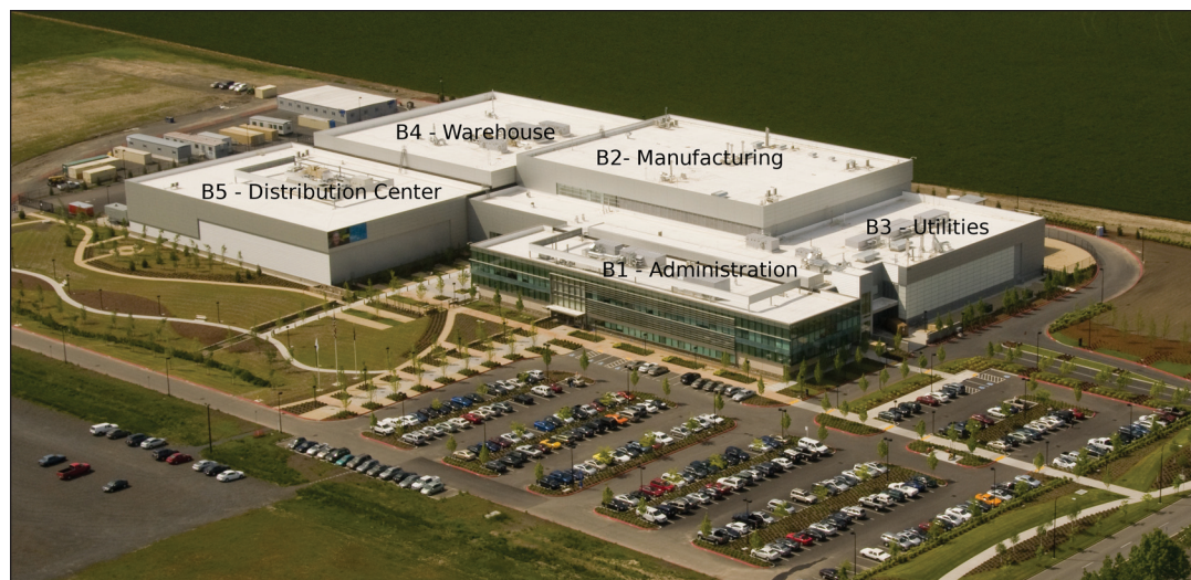
Figure 1. The construction sequence of the facility was governed by completing B5 first, followed by B4, utilizing the high bay space for material storage followed by the manufacturing, utility, and administration buildings.
