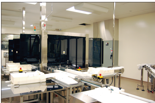
Figure 5. Inspection lines are visually connected to the fill suites to ensure ease of communication. Within the inspection suite, there is the capability for both automated and manual inspection.
